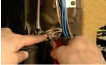
6. Interrupt compressor (or compressor contactor) switching wire. This is the cable through which the thermostat tells the compressor to run or stop.
