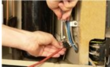
7. Route this wire through the Aircosaver (i.e. the Aircosaver is now logically in series with the thermostat). Connect power to the Aircosaver.
